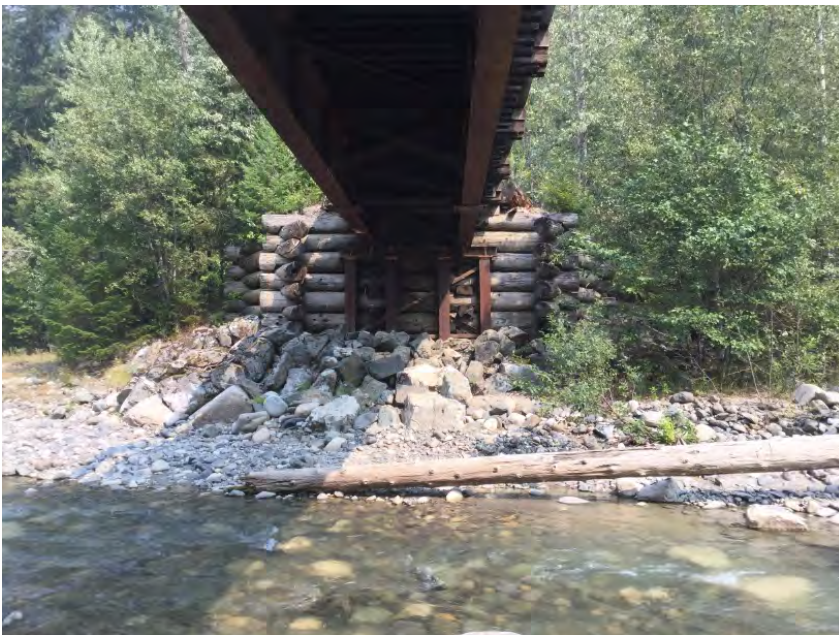
Right Bank Abutment when facing downstream
