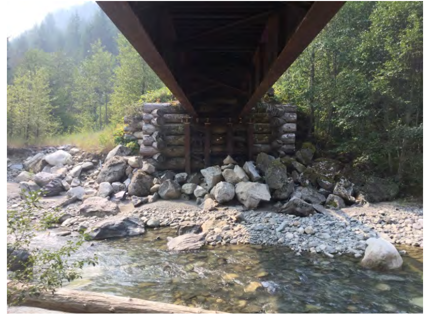
Left Bank Abutment when facing downstream
