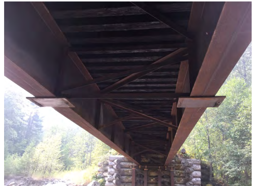
Old bearing plates still visible
